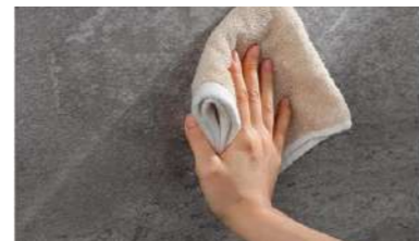
01. Wipe the wall clean with a towel
